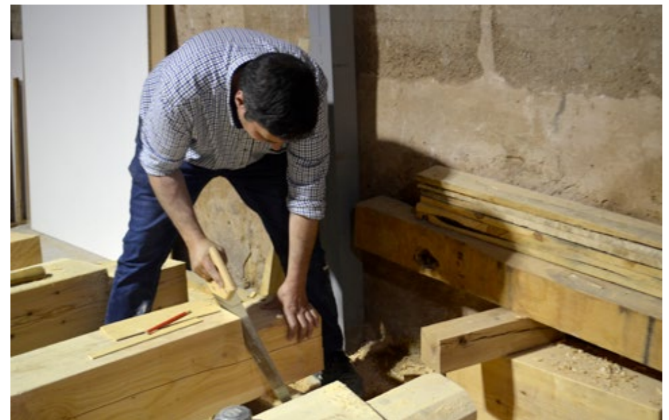
Construction of the wooden frame that secures the milling machinery
