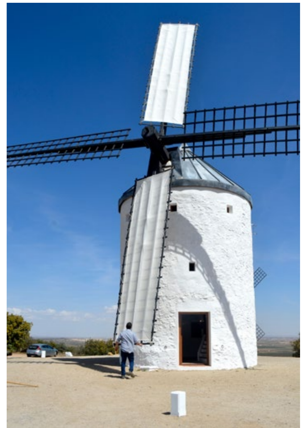
Fitting of sailcloth on the sails of the mill in Puerto Lápice
